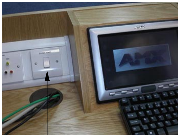
Desk Power Switch
