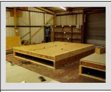
Fig 2: Floor systems supported on shallow wall panels
